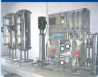
PLC Based RO System - Full SS
