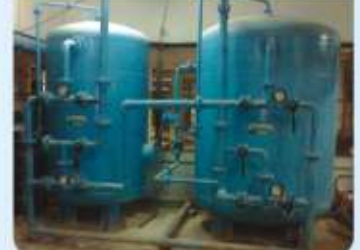
Multiple Filtration & Softener Plant - MSRL
